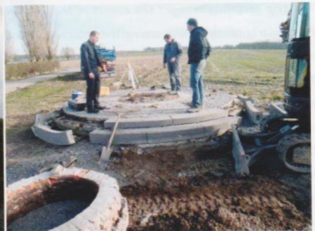
Dismantling the Memorial
