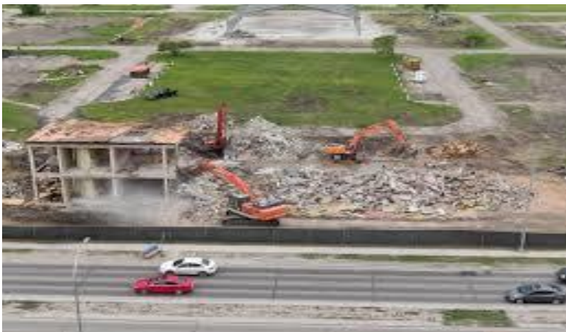
Demolition of the Lecture Training Building.
