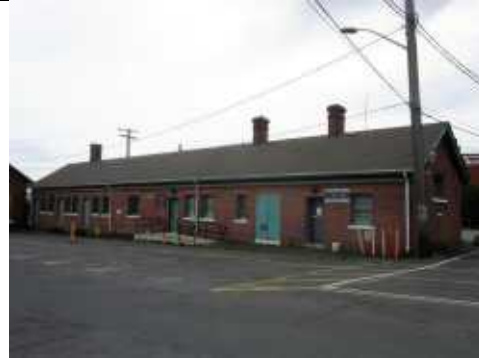
“ARLEUX BUILDING – 2019 – Band, AAP and Kitchen Stores – 1994”
